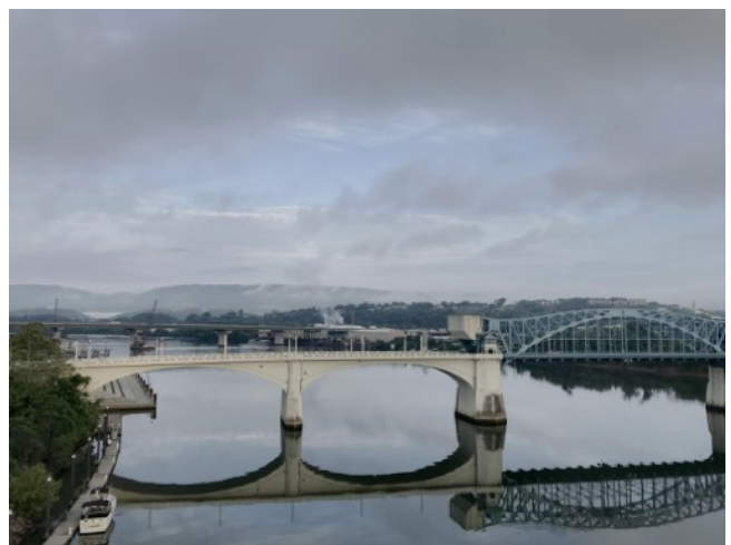
The view from the opposite side of the bridge, looking west.
